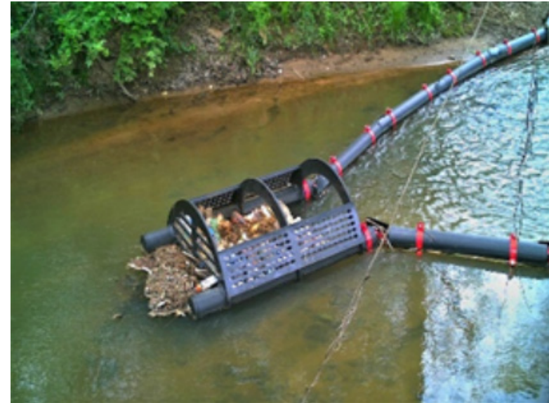
Photo Credit: Storm Water System. An example of a litter trap.
