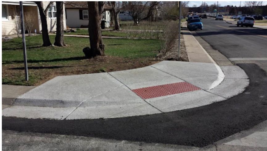
Photo Credit: Business Though. An example of safe, gradient sidewalk ramps into intersec-
